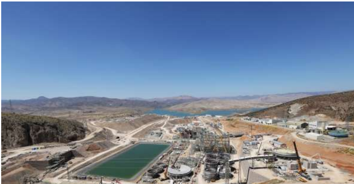
Overview of the Project Site
