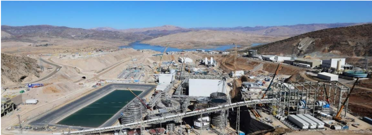
Overview of the Project Site
